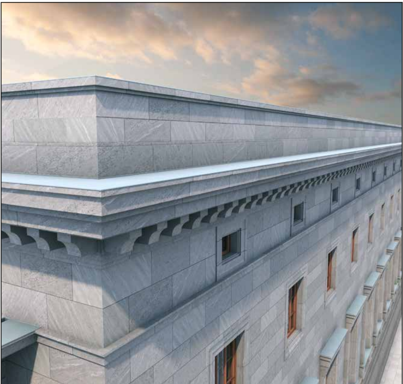
Fig. 63 The attic parapet at the western corner of the Central Building
