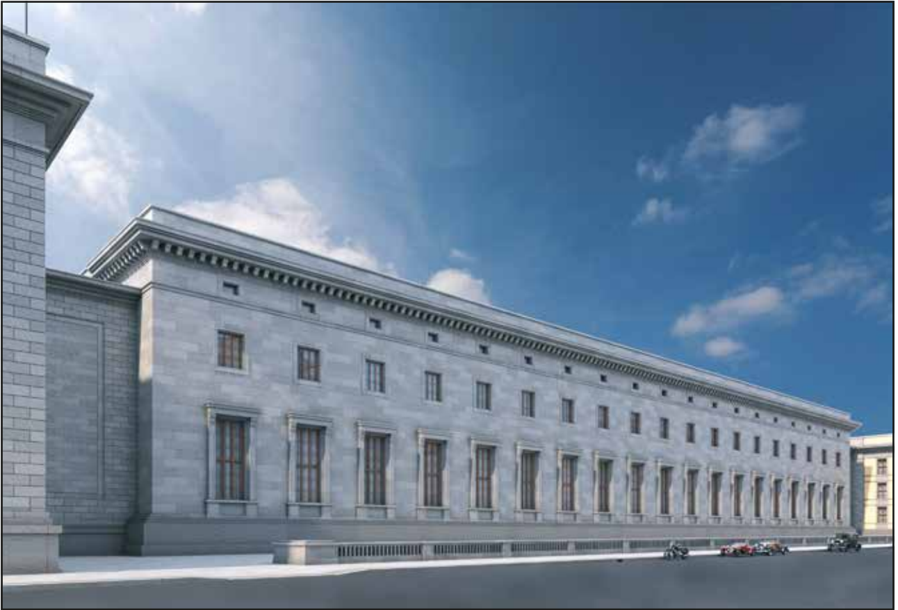
Fig. 58 The design of the Central Building created the illusion of ceiling heights that did not correspond to reality
