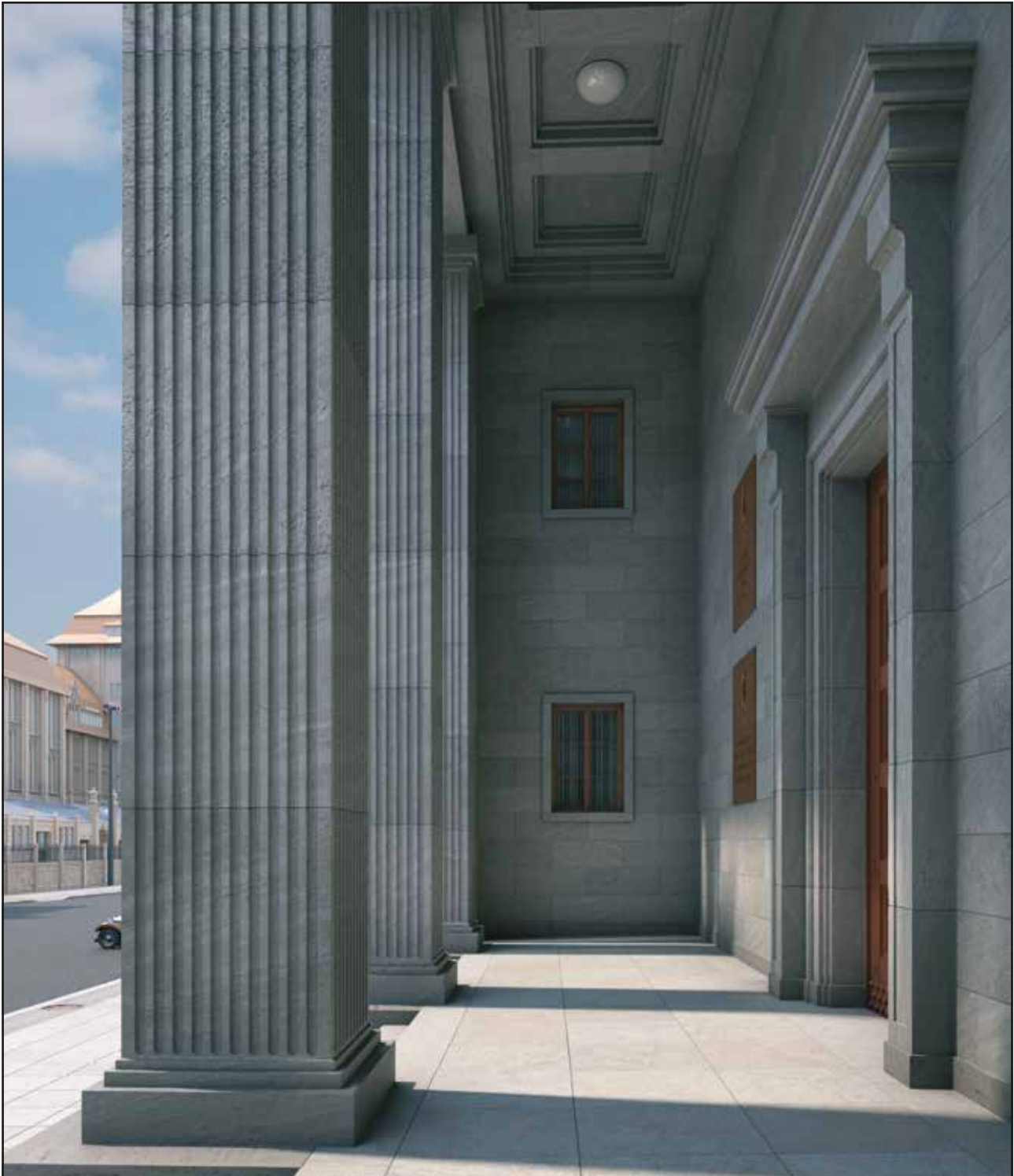
Fig. 95 View of the western narrow side of the portal's vestibule
