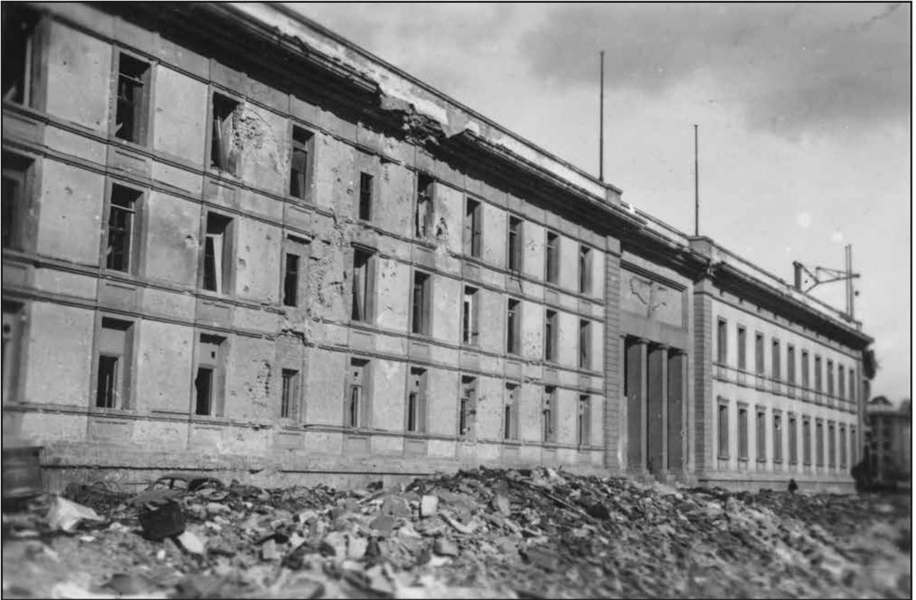
Fig. 131 This photo shows the partially bricked-up damage to the window openings (1945)
