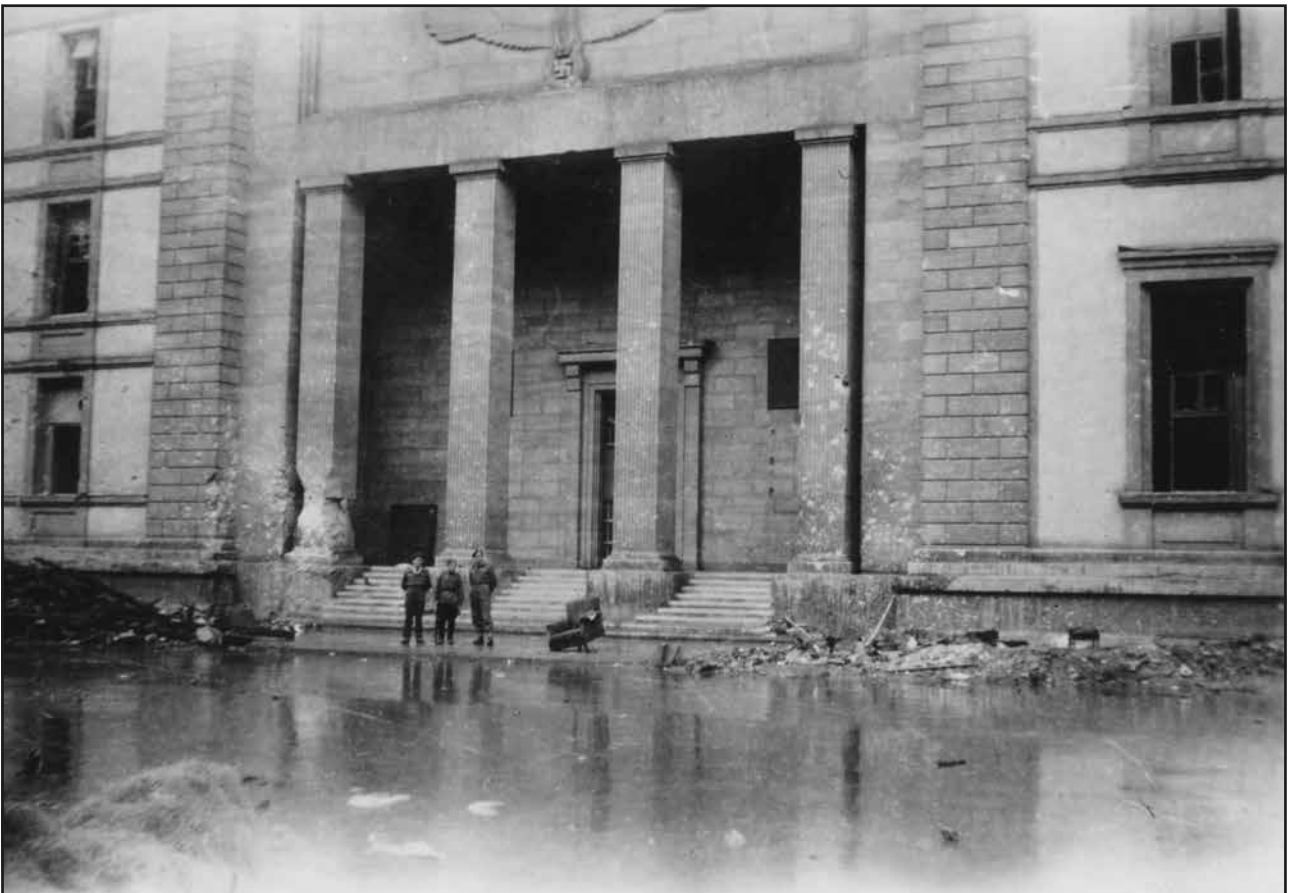
Fig. 132 The Presidential Chancellery portal damaged by artillery fire (1945)
