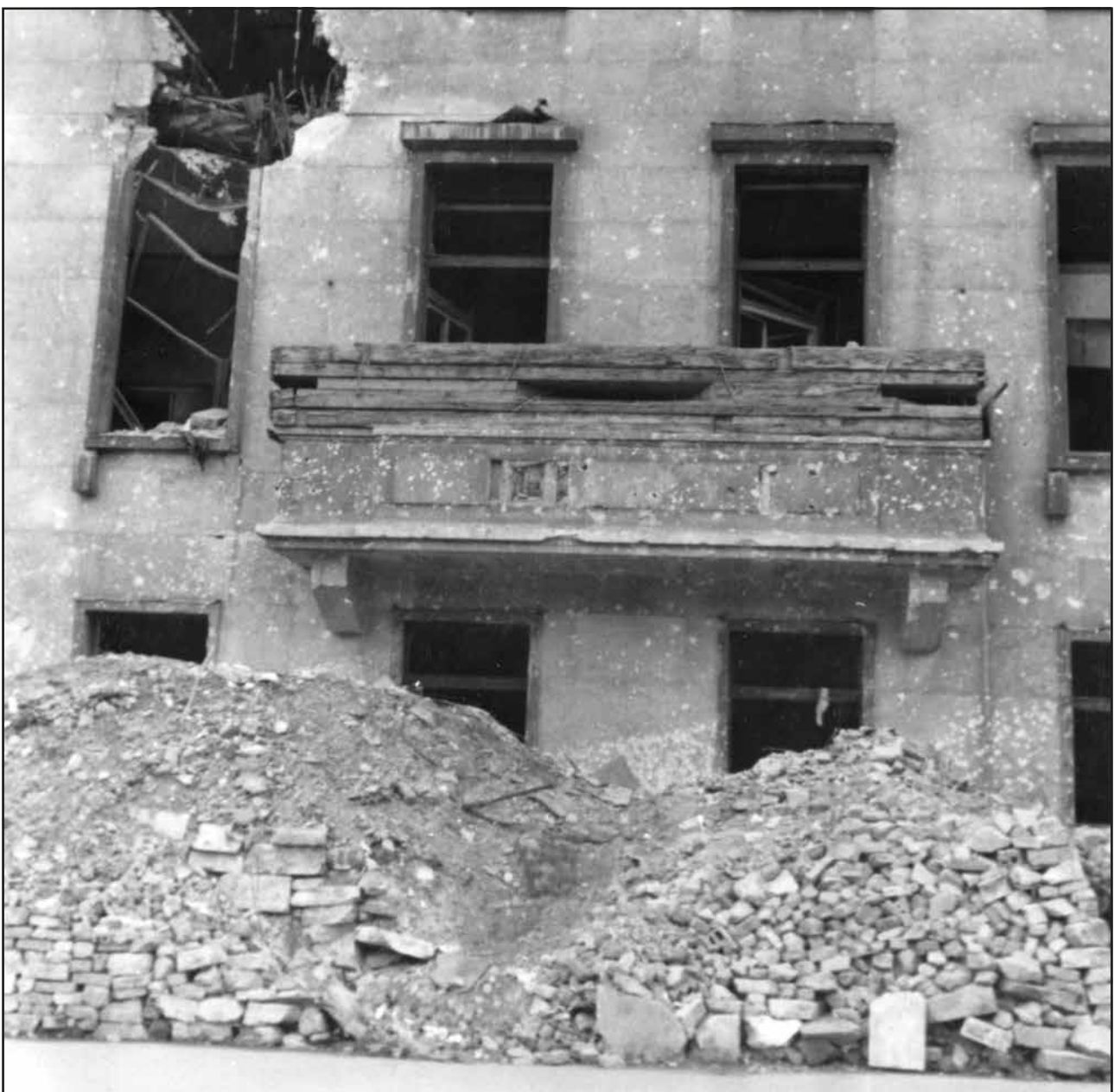
Fig. 104 This photograph, taken on July 1, 1945, shows the Führer balcony reinforced with wooden planks
