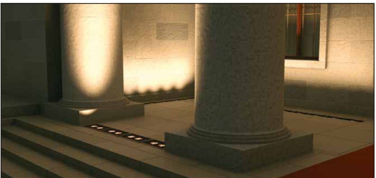
Fig. 109 In the portal, the spotlights were placed in the floor in front of the walls and between the columns
