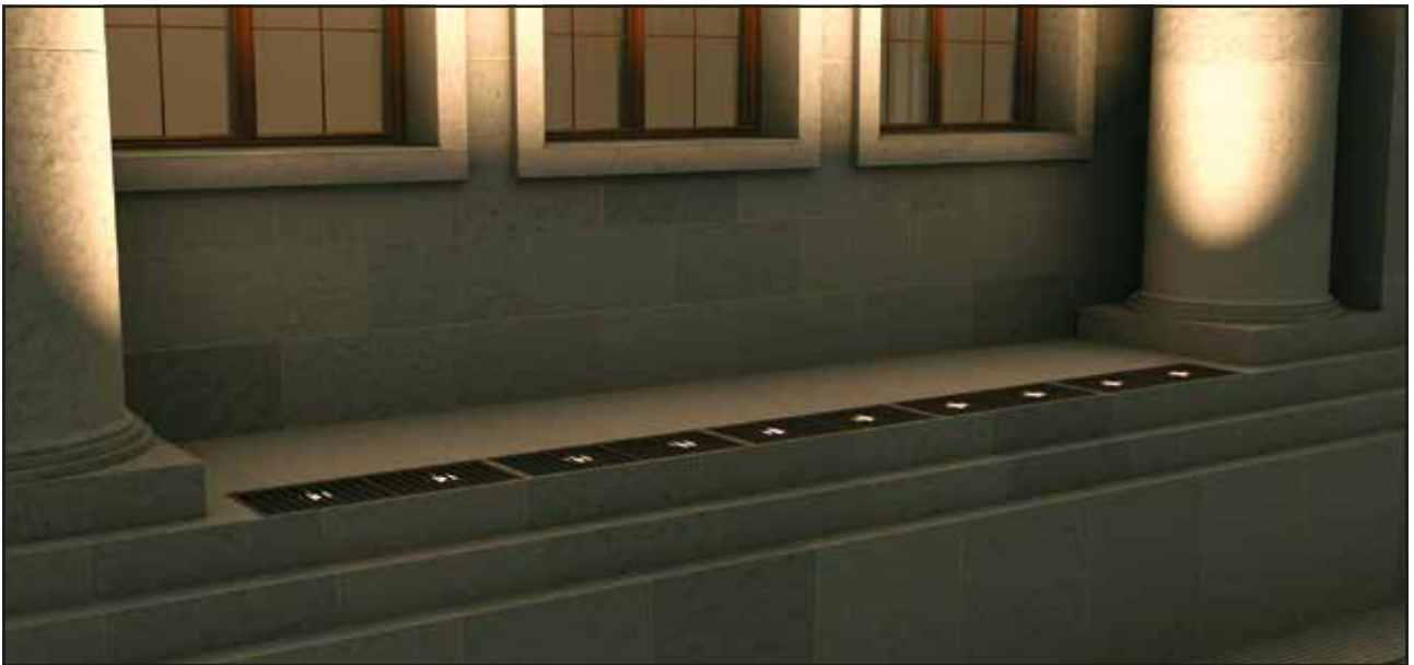
Fig. 108 Speer integrated the spotlights into the portal niches of the longitudinal facades
